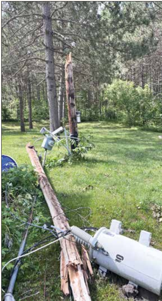
Damaged transformer and meter pole.
